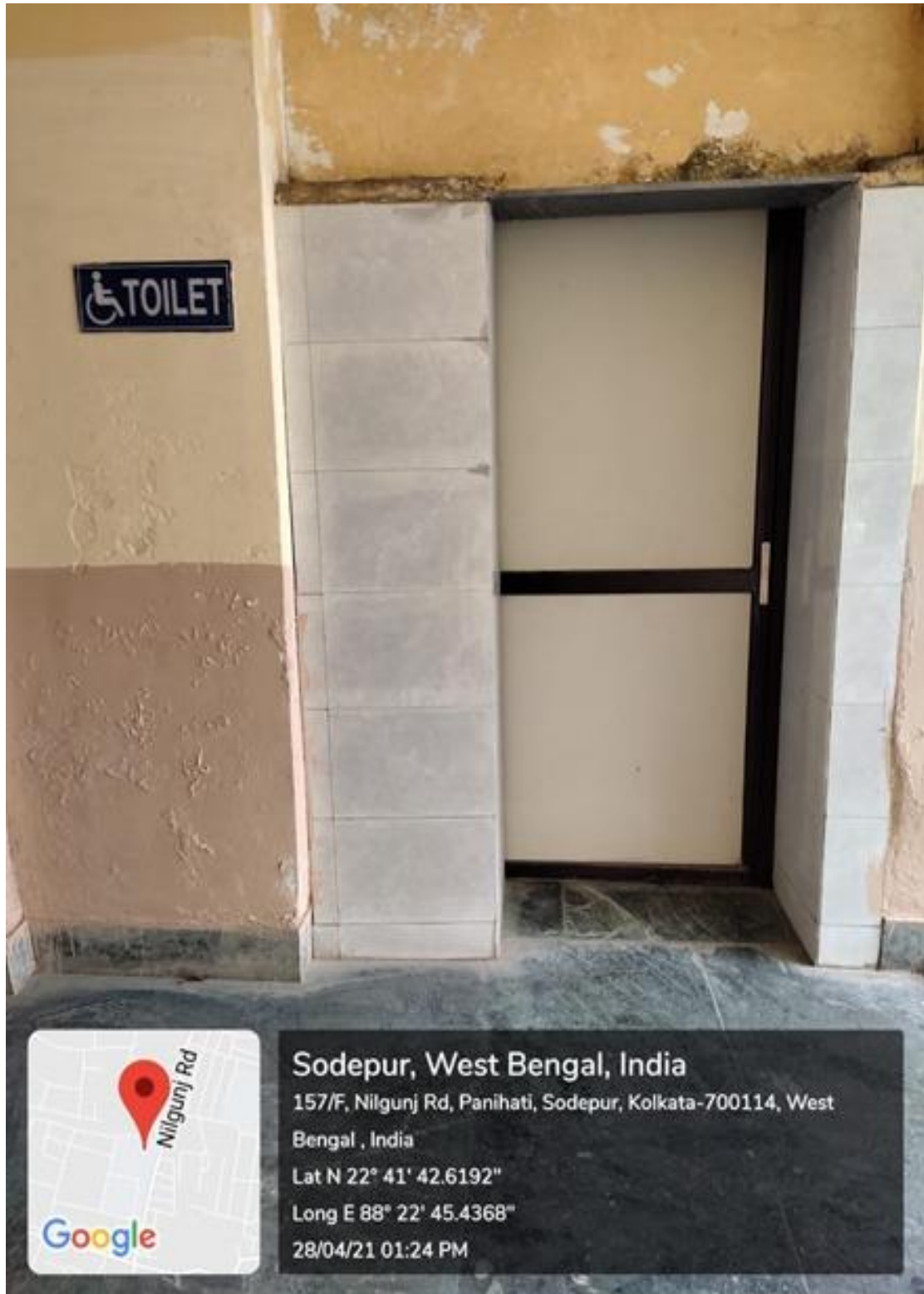
Toilet for Disabled Staffs
